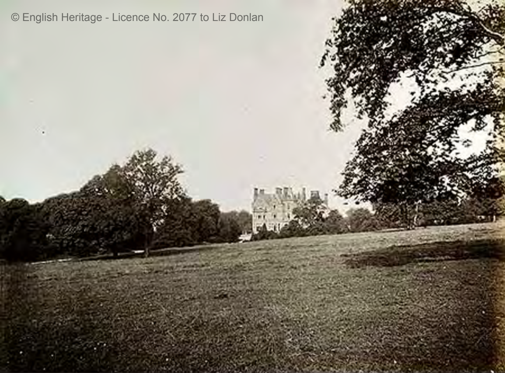
Distant view of the entrance front of the Hydro from the park. Photo taken 5th September, 1889
